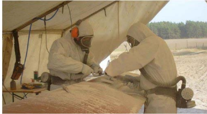
Figure 1: Repair lamination of wind generator wings, KOOP
