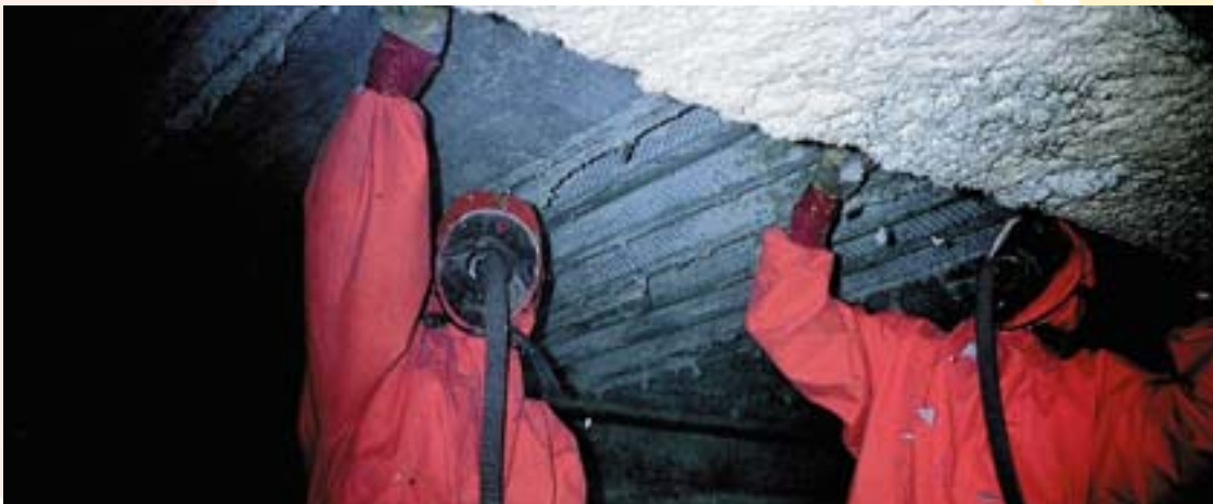
Courtesy of OPPBTP, France
