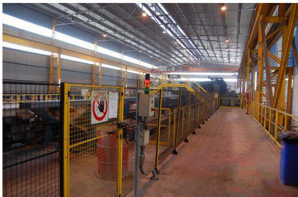
Figure 3. Installation of metal fences
