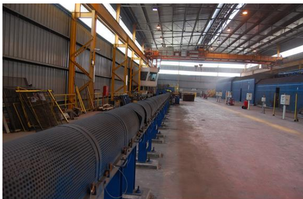
Figure 1. View of the path of the production line already covered
