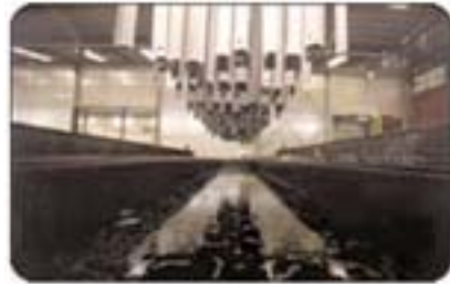
The activated pickling system
