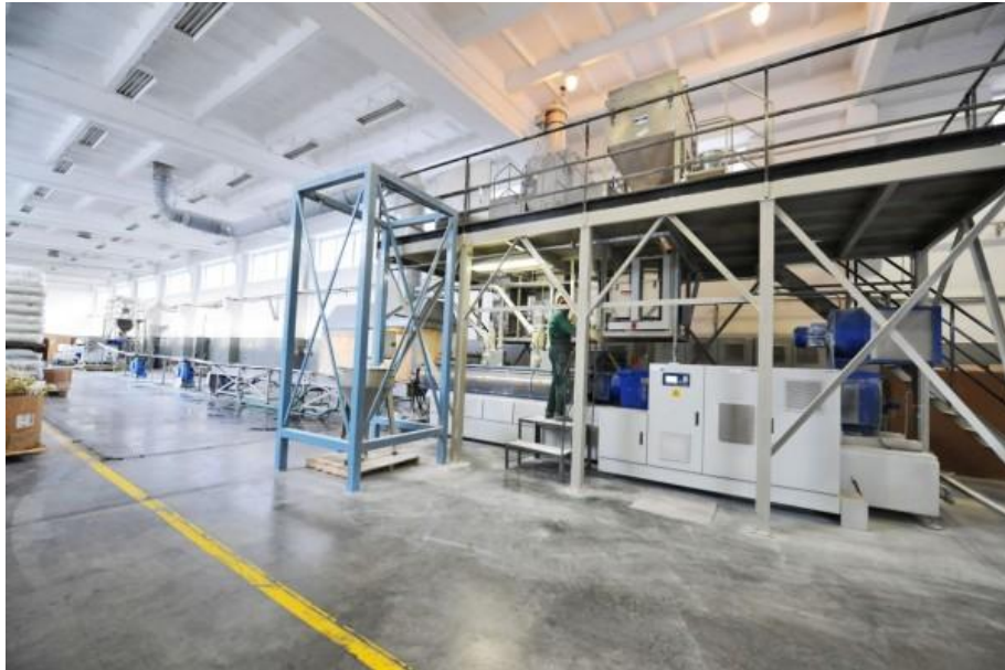
Figure 3: Manufacturing room – protection measures: sealing of the production line and ventilation of the manufacturing room.
