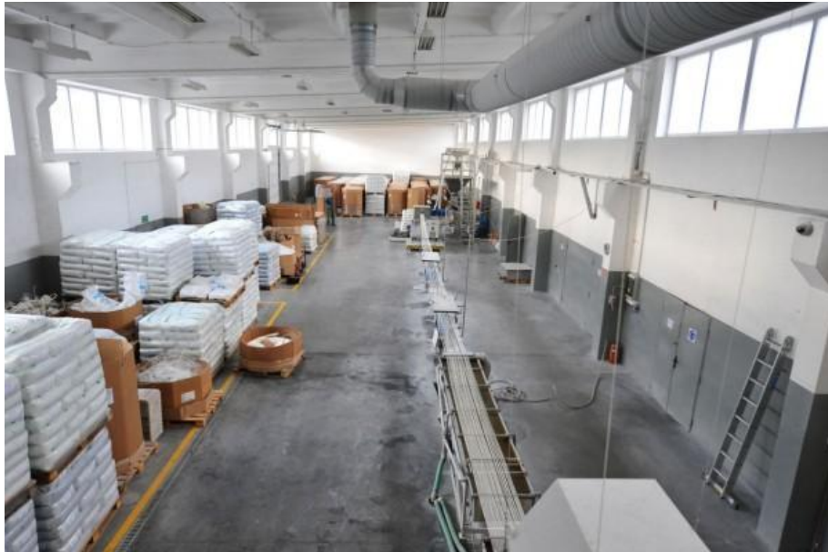
Figure 1: Raw material warehouse – protection measures – ventilation
