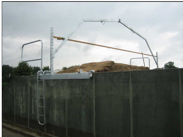
Figure 1: Mobile railing (Source: G. Lange, German statutory accident insurance for agriculture).
