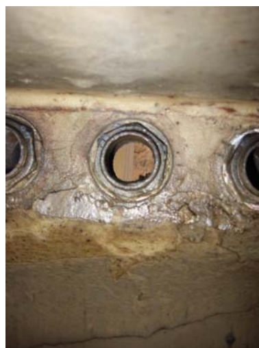
Picture 2. Sediment and debris on walls and bottom of water tank
