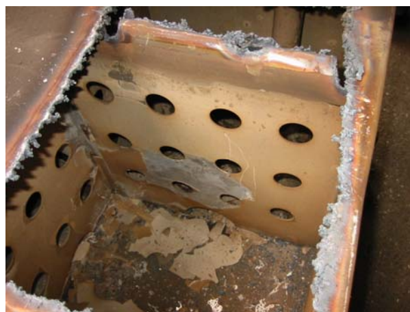
Picture 1. Visual inspection of a water tank
