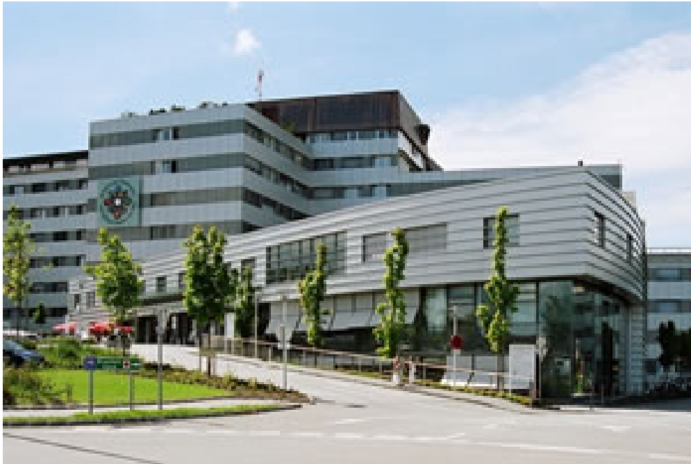
Picture 1: Barmherzige Schwestern Ried Hospital, new building (Bauteil 6)
