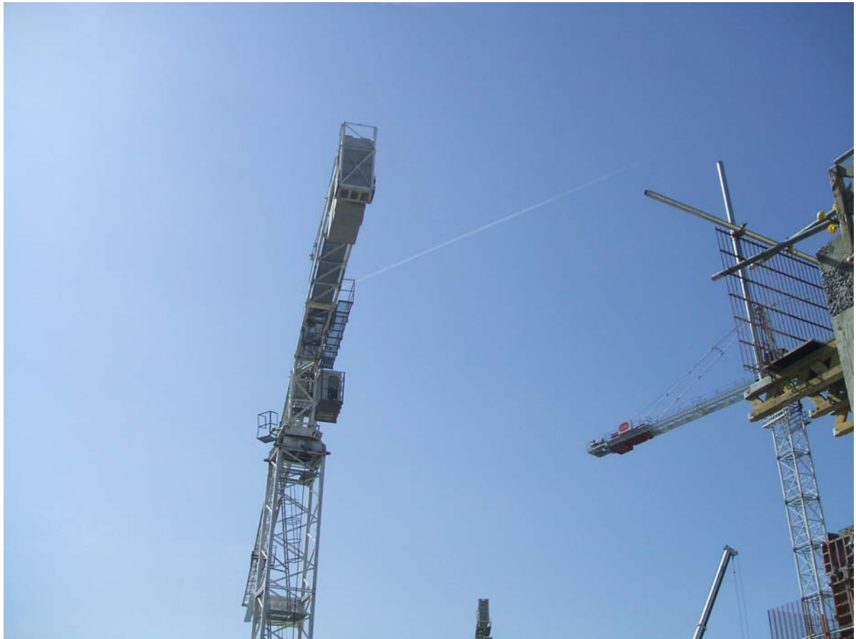
Figure 1. Multiple tower cranes at a construction site
