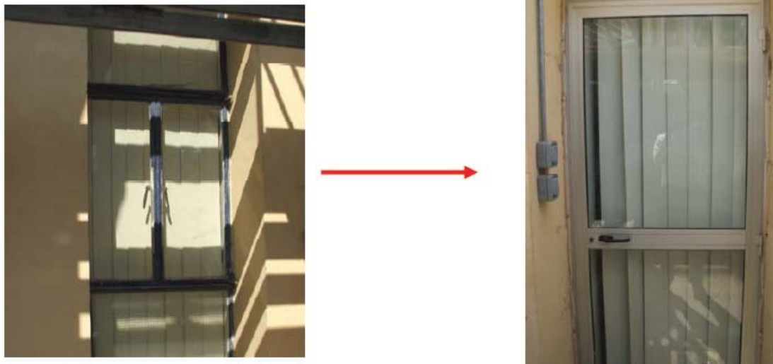
Fig.4 Access to external technical area was originally through a window which was converted to a door for easier and safer access
