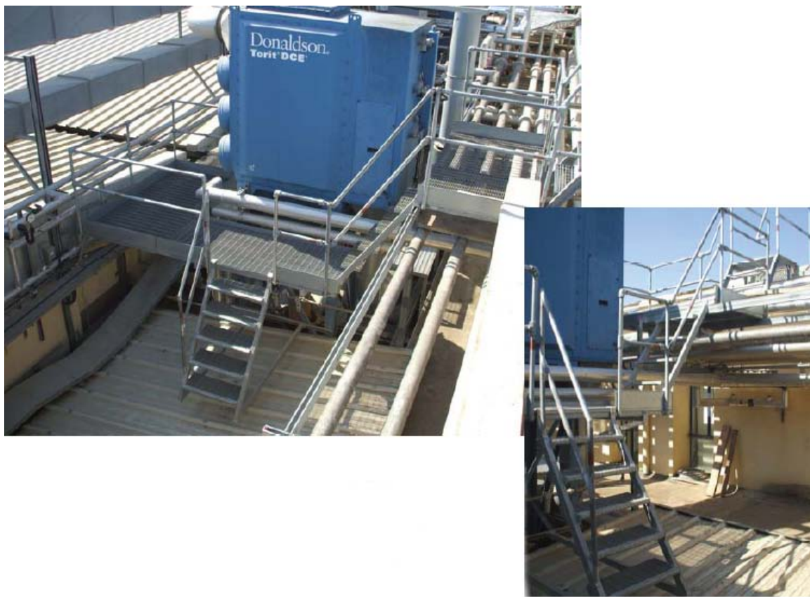
Fig.5 Installation of a working platform around the Dust Collector improved accessibility and rendered the preventive maintenance job safer
