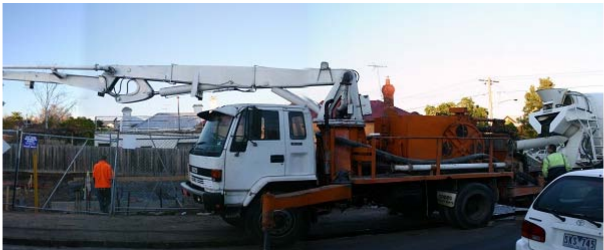
Fig. 1 Truck-mounted concrete pump, source: Wikimedia. When driving, the distribution booms are folded and rest on the loading area.
