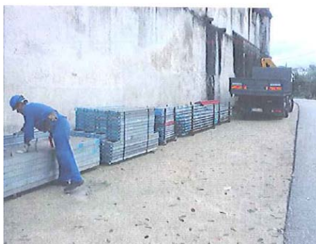
Picture 4. Offloading scaffolding outside the monument
