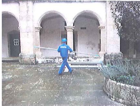
Picture 5. Difficulties in accessing the work areas meant materials had to be moved by hand
