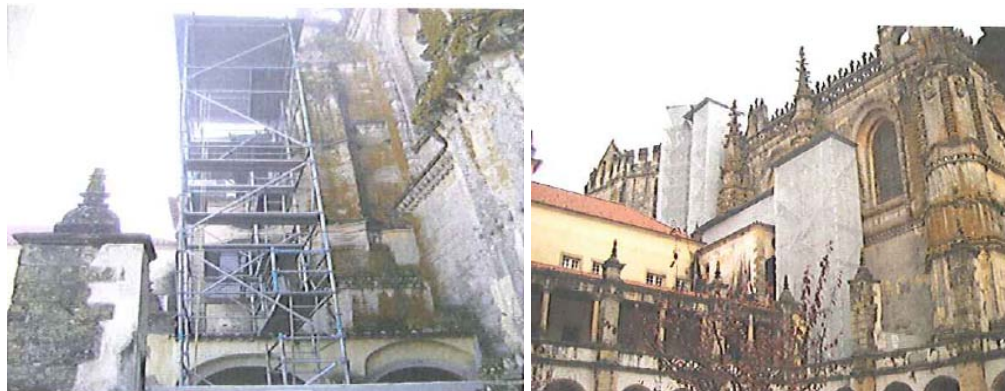
Picture 3. Scaffold during and after installation on the manueline façade
