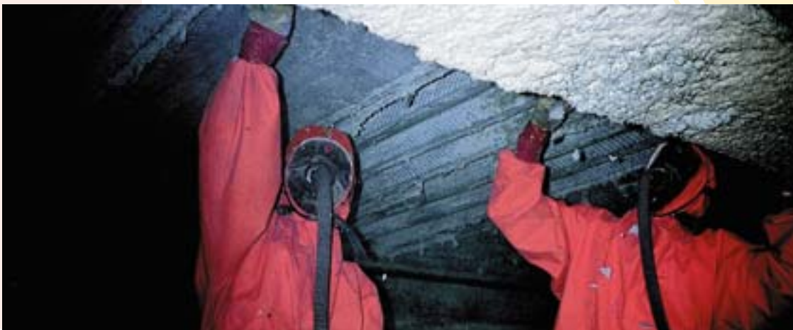
Courtesy of OPPBTP, France
