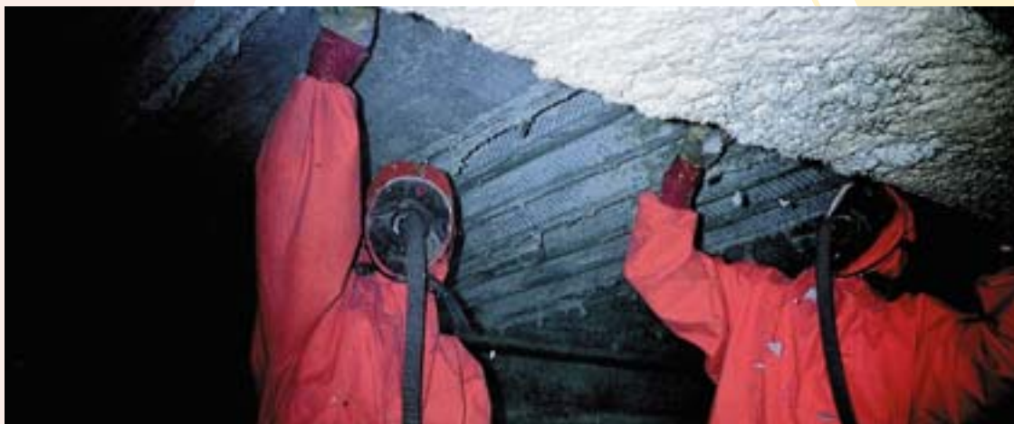
Courtesy of OPPBTP, France
