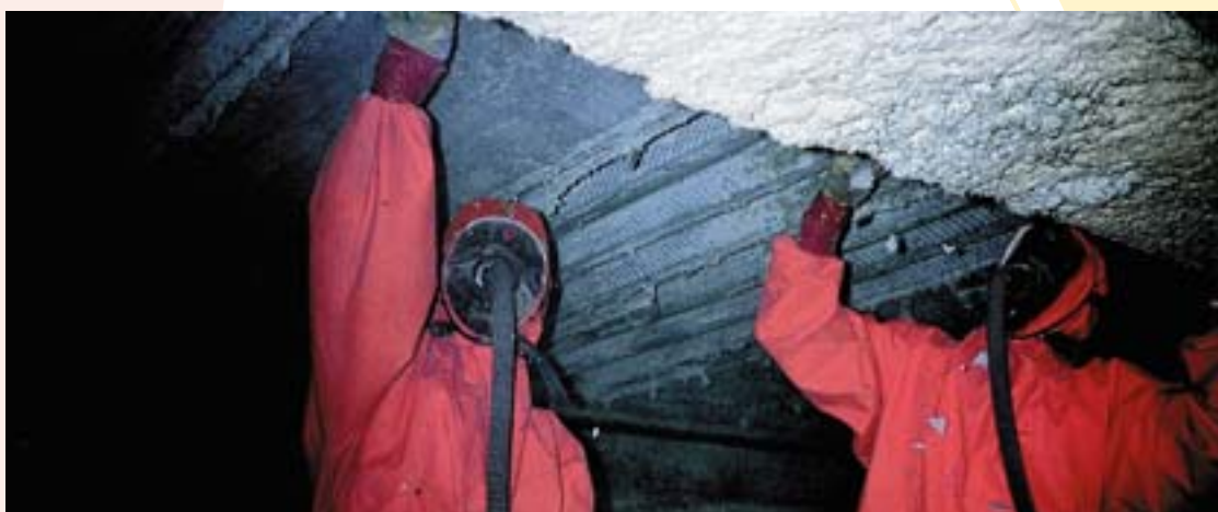
Courtesy of OPPBTP, France
