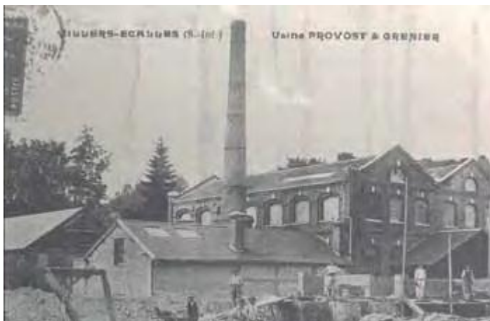
Picture 1: Old photograph of the “Prevost et Grenier” weaving mill that was purchased in 1959 by Ferrero
