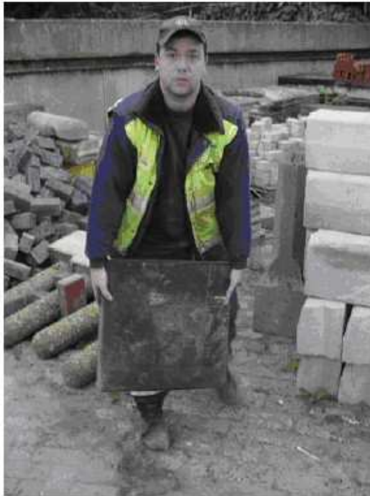
Figure 1 A 60 kg 500 × 500 × 80 mm tile that is very fragile. The elongated concrete stones and paving bricks exceed the maximum 4 kg weight. The other bricks weigh less than 4 kg.
