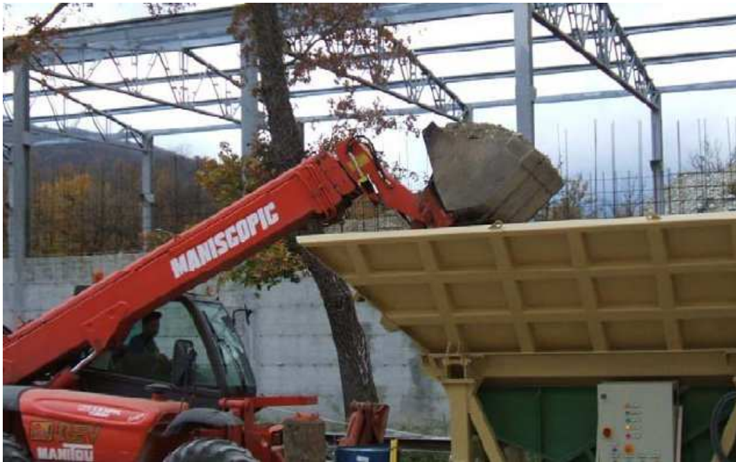
Figure 6 Use of a mechanical loader to move material to the hopper
