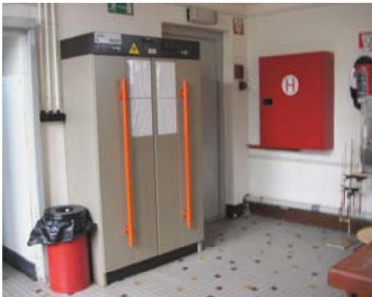
*Security locker for flammable products stored inside the laboratory*
