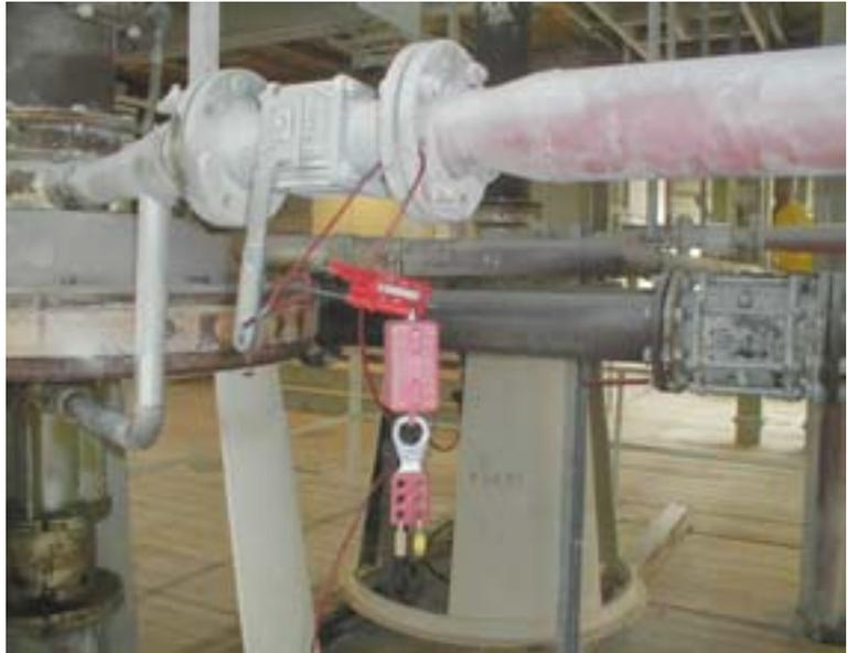
*Lockout on a pipe to prevent unintentional release of hot steam. The master lock in the red box blocks the clip. The master lock cannot be removed before the two workers have removed their personal keys*
