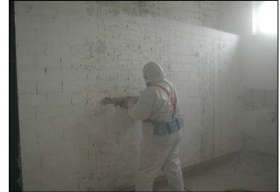
Chipping off without extraction.
