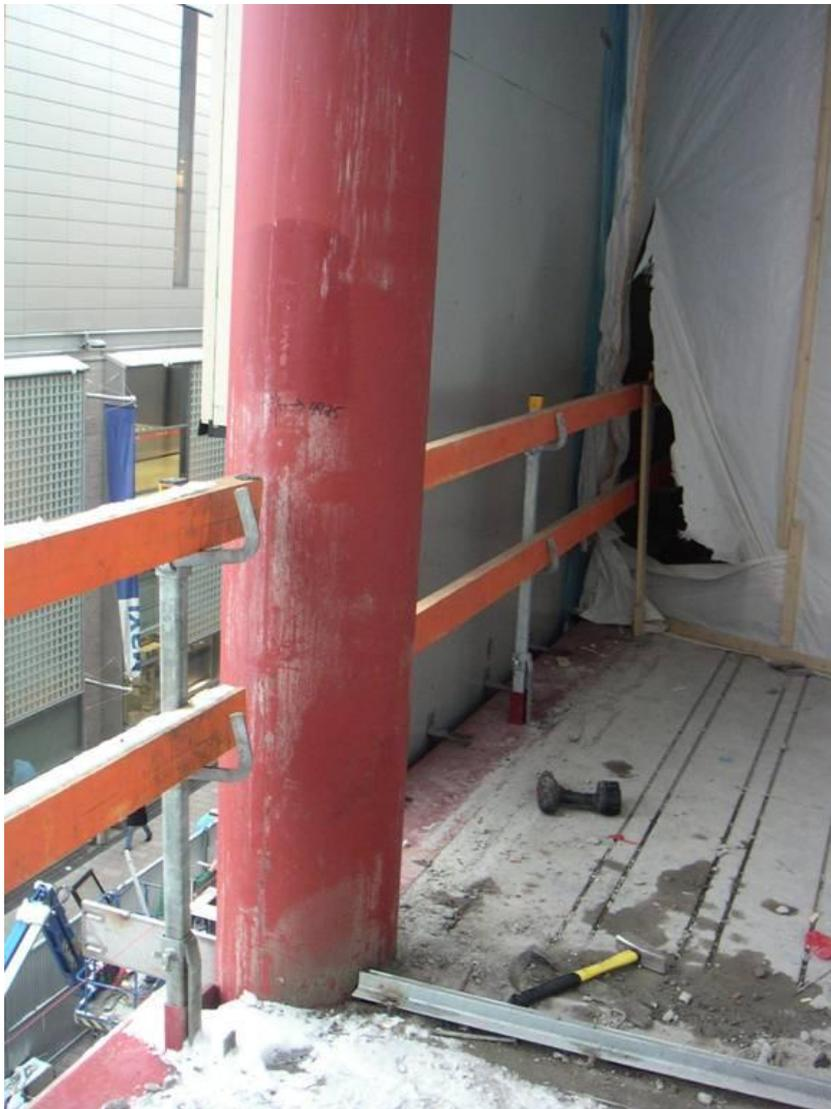
Picture 2: The safety rails were installed before the installation of wall elements. Source Henri Mämmi NCC, copyright NCC.
