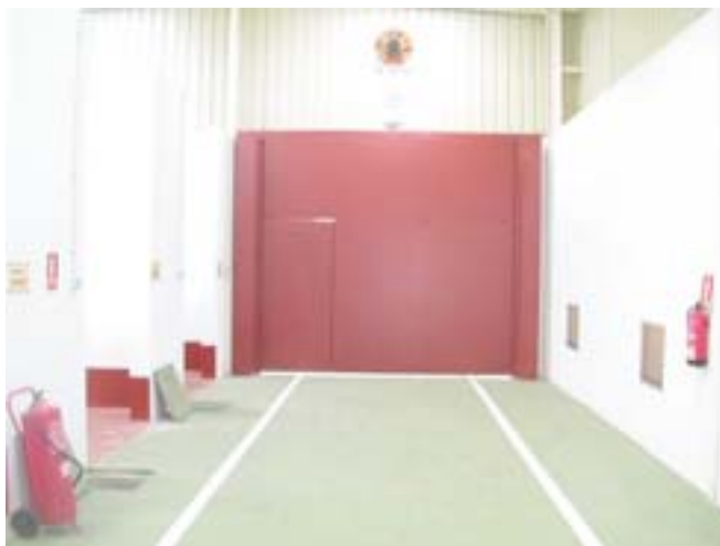
Interior of the main area of the storage facility. On the left are the different storage modules. N.B.: there is both forced ventilation installation (top centre) and natural ventilation (bottom right)
