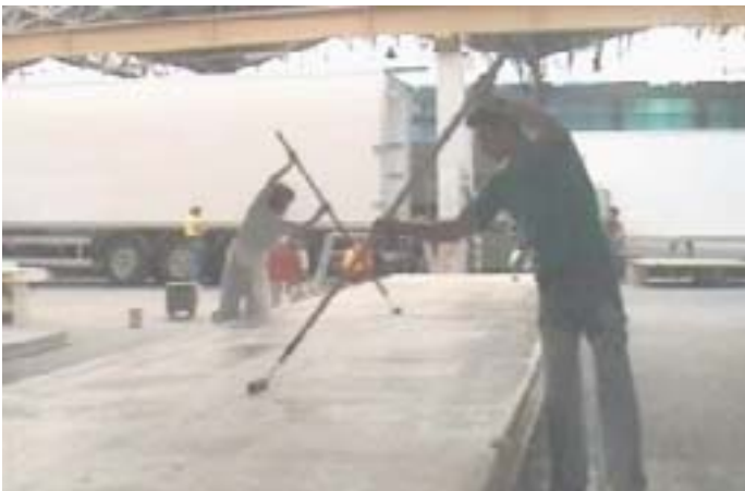
Before: resin spreading with rollers
