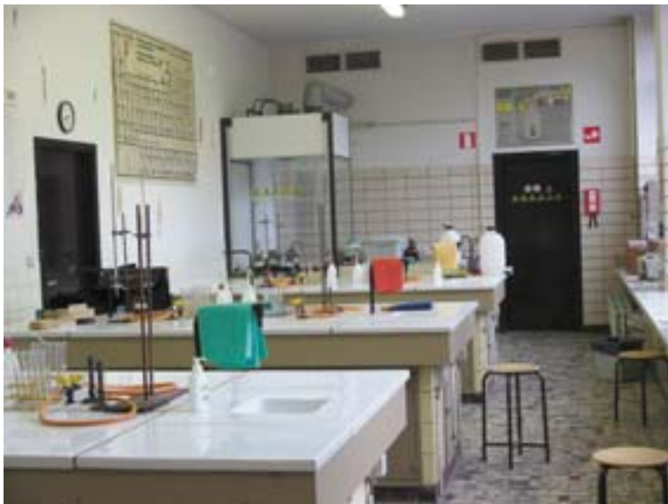
School laboratory with an air extraction device
