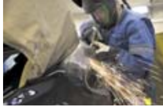
Before: cross-grinding without the integrated extractor device
