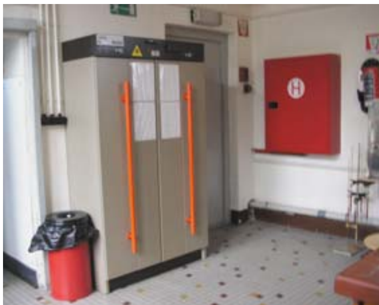
Security locker for flammable products stored inside the laboratory
