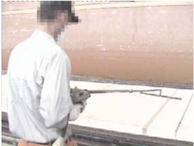
After: application of polyurethane glue
