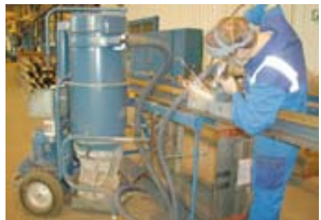
After: spot extraction for insulated rail joint grinding
