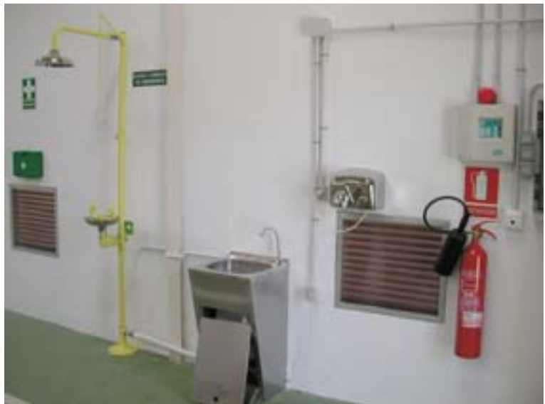
From left to right: first-aid kit, eye wash, showers, sink and hand drier, CO 2 extinguisher and alarm
