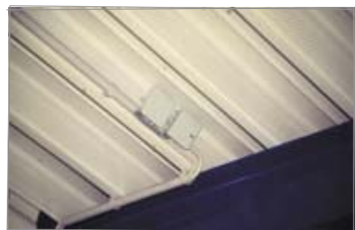
Figure 5: Close-up of the sound-absorbent profiled-steel ceiling
