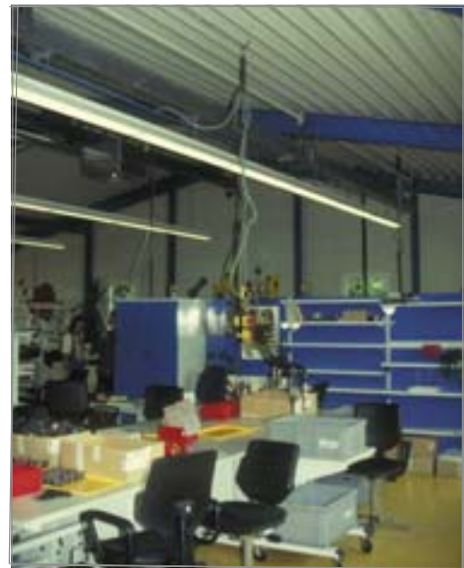
Figure 4: Metalworking unit with sound-absorbent profiled-steel ceiling
