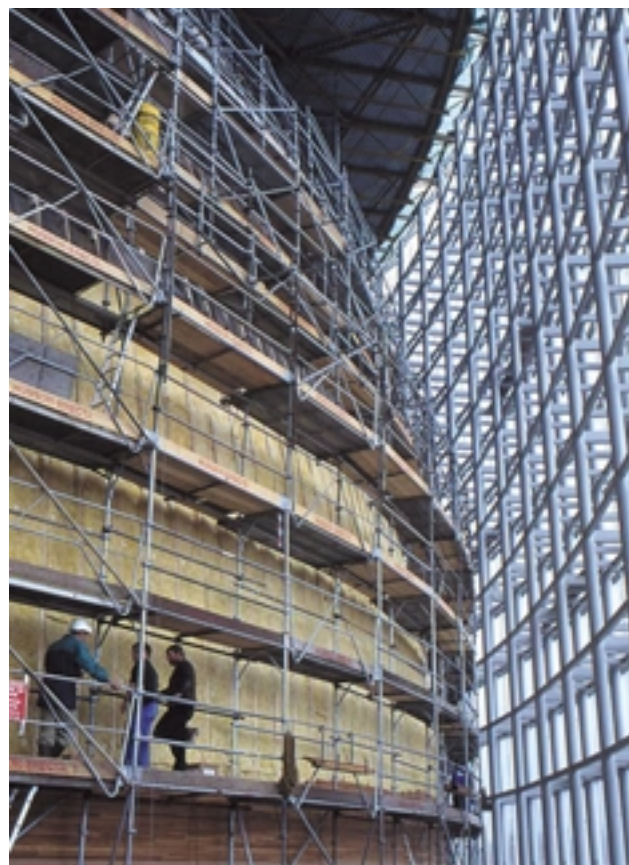
Scaffolding in the European Parliament construction site in Strasbourg.
