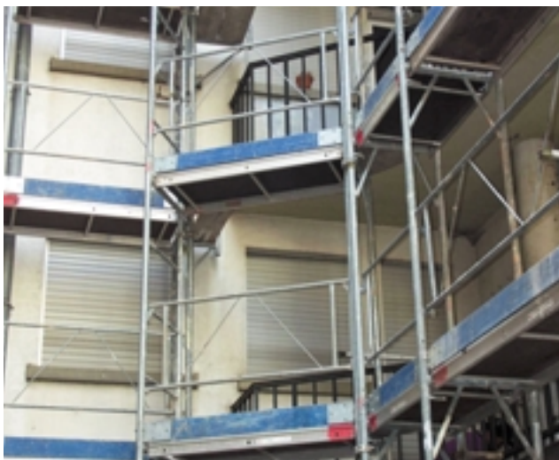
Scaffolding in the European Parliament construction site in Strasbourg.
