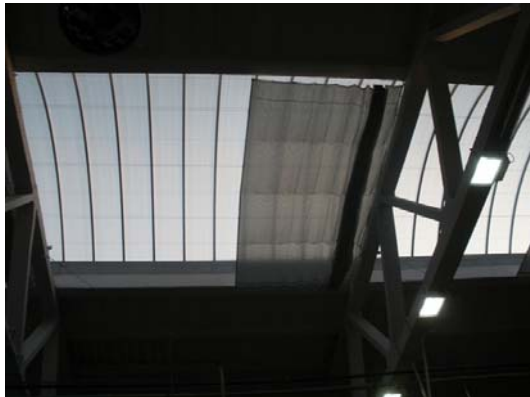
Figure 9. Use of safety curtains to prevent penetration of light and heat
